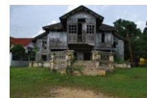
Fig. 2. Dilapidated conditions of the building
