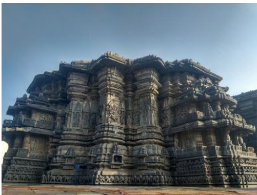
Fig.9. Stellate design of the walls and the roof
