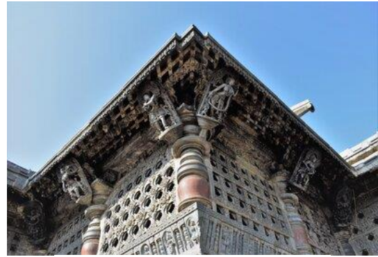
Fig. 10. Mounted bracket figures on the eaves.
